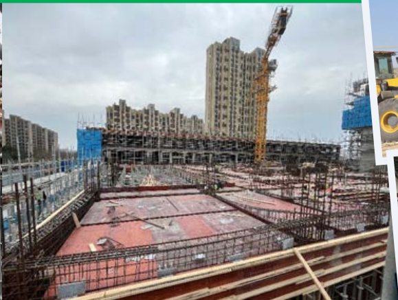
Traditional usage of New Zealand lumber, as concrete formwork
