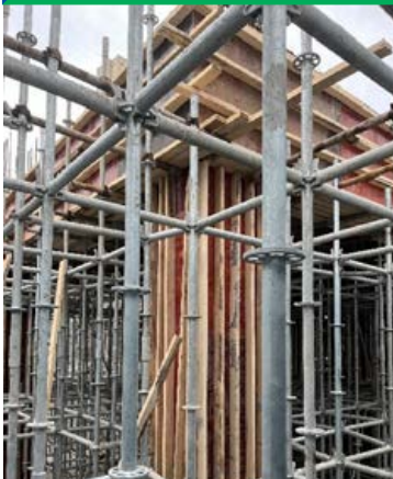
Traditional usage of New Zealand lumber, as concrete formwork
