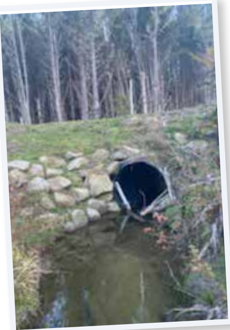
Figure 8: Large rocks tightly packed around culvert inlet provide protection
