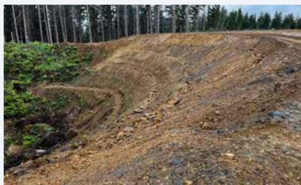
Figure 4 Jilesen: Completed fill benches
