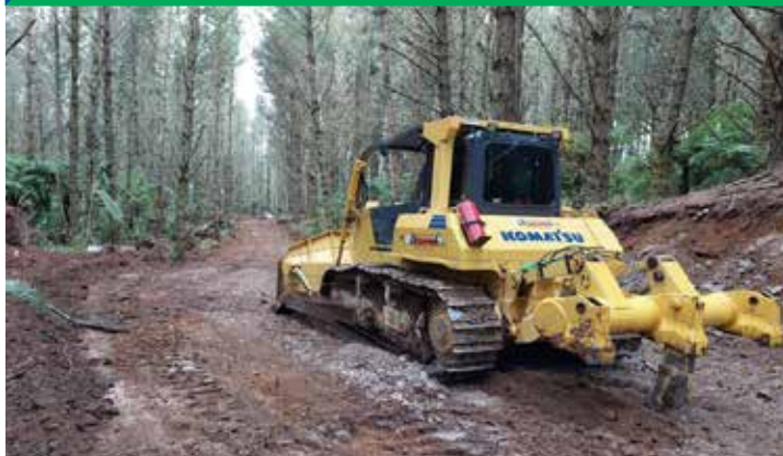
Figure 1 Archer bulldozer forming a new road
