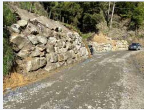
Figure 11 Retaining boulder wall neatly stacked along with drainage to prevent further movement
